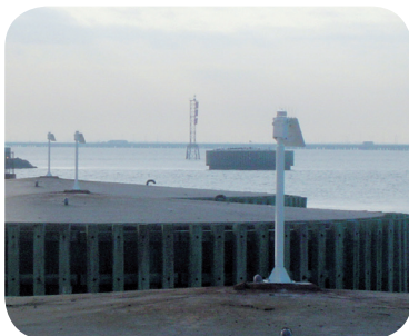
Sealite SL-23 marine lights mark the famous Sunshine Skyway Bridge, Tampa, Florida
