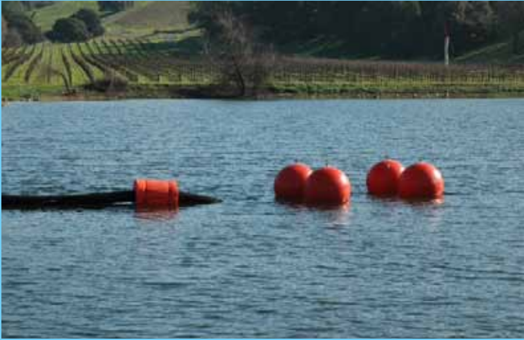
Courtesy of: Lodi Irrigation/ Submersible pump and pipeline suspended by Rotonics Float Balls & Pipe Floats
